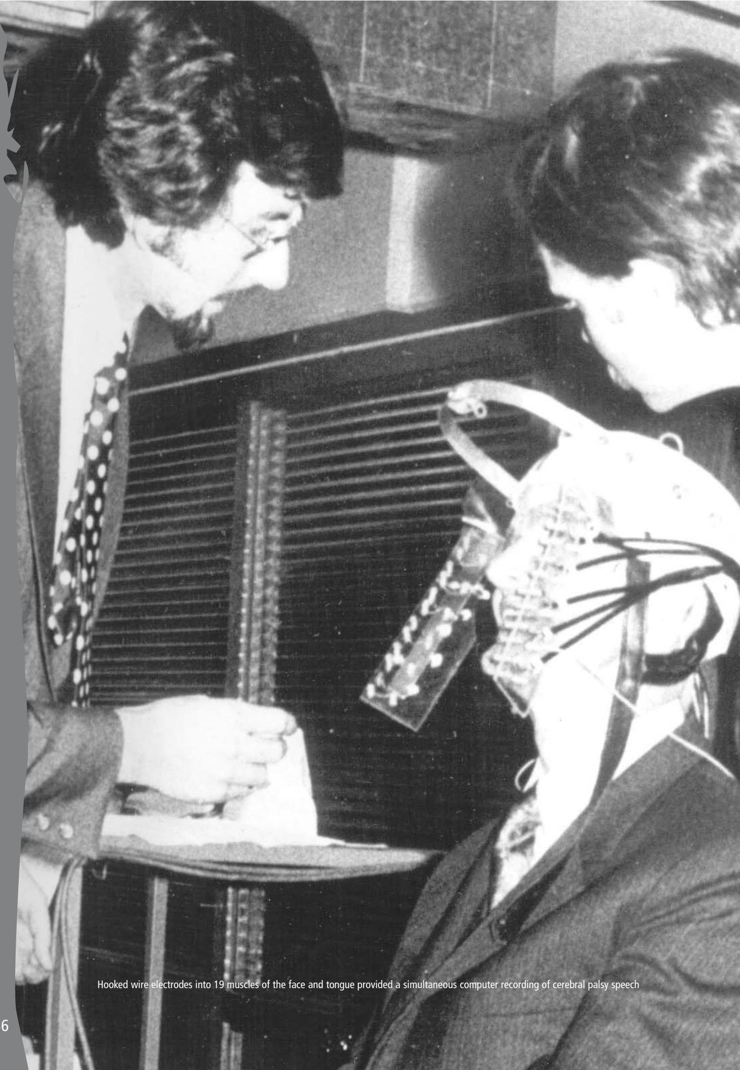
Hooked wire electrodes into 19 muscles of the face and tongue provided a simultaneous computer recording of cerebral palsy speech
